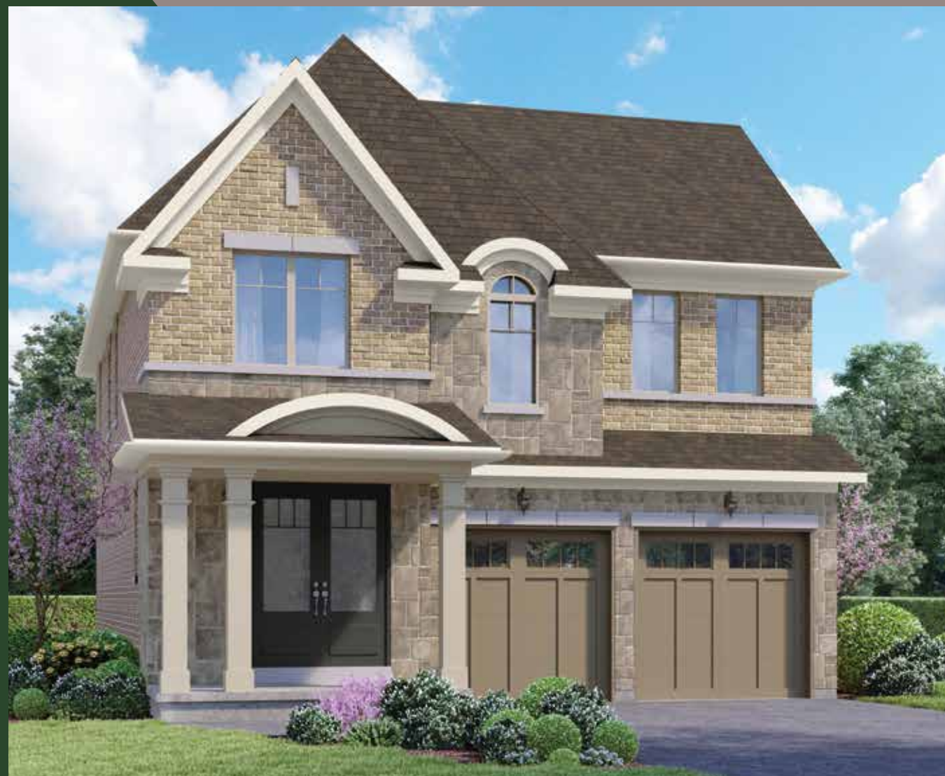
ELEVATION A ELEVATION B 2451 SQ. FT. 2434 SQ. FT. ADD 738 SQ. FT. FOR ADD 738 SQ. FT. FOR OPTIONAL FINISHED BASEMENT OPTIONAL FINISHED BASEMENT
